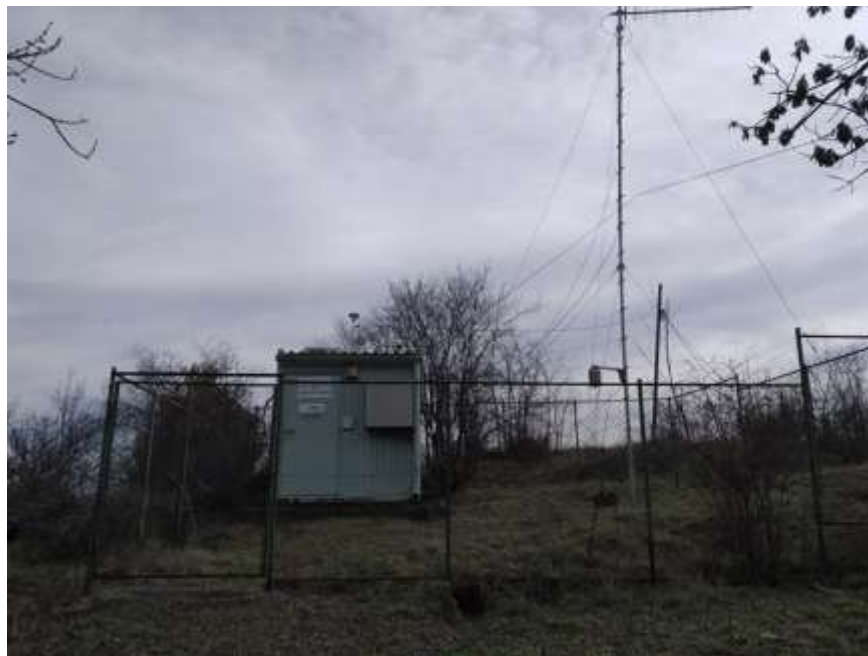
Figure 2 Automatic monitoring station – Gazi Baba
