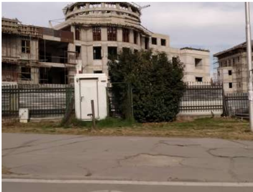
Figure 3 Automatic monitoring station – Rectorate
