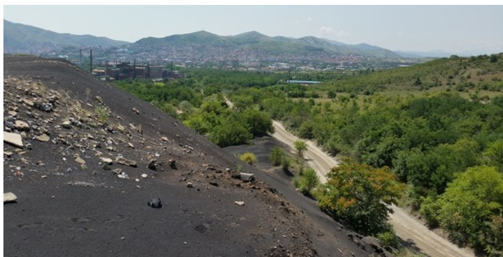
Fig. 1. Metallurgical waste dumps after processing of lead and zinc concentrates in Veles, Republic of Macedonia (photo: R. Šajn)
