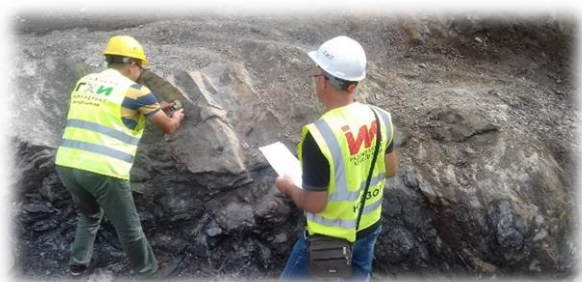
Fig. 1. Geological mapping of foundation pit at the Otinja dam
