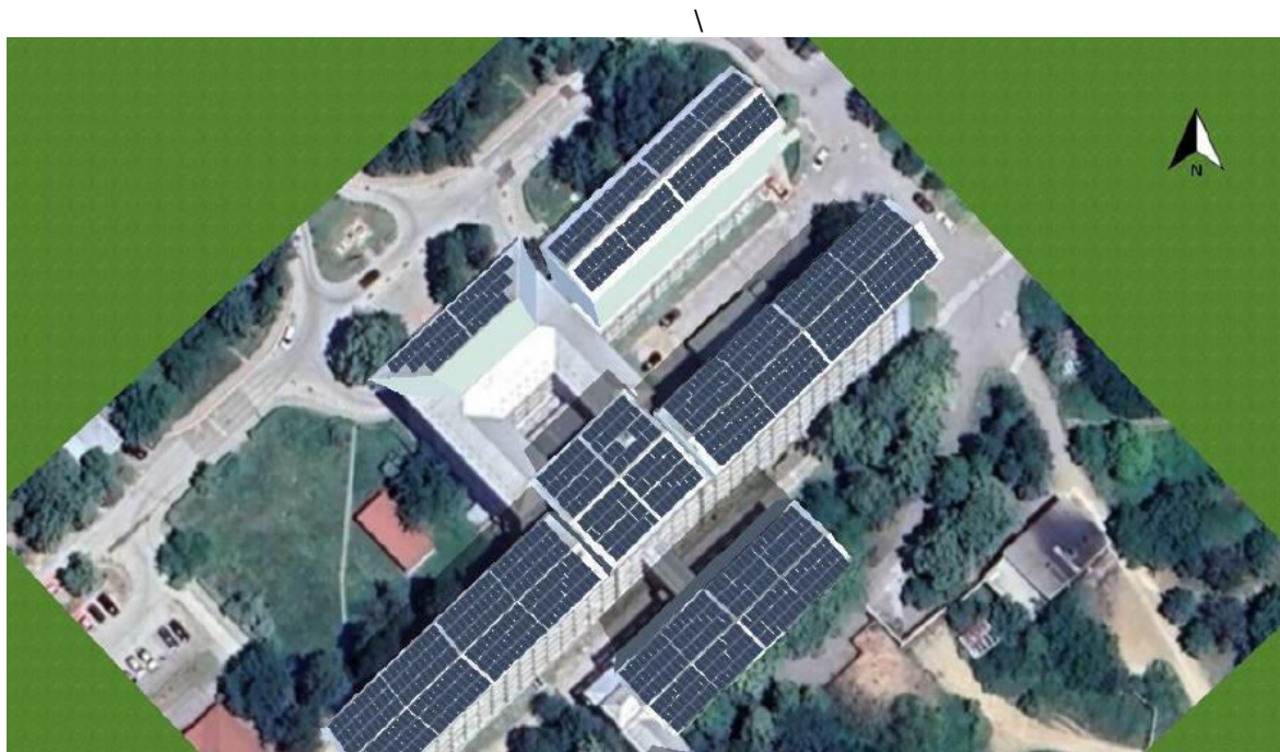
Figure 1. Example of a designed rooftop PV system in Bitola (PV*SOL premium visualization)
