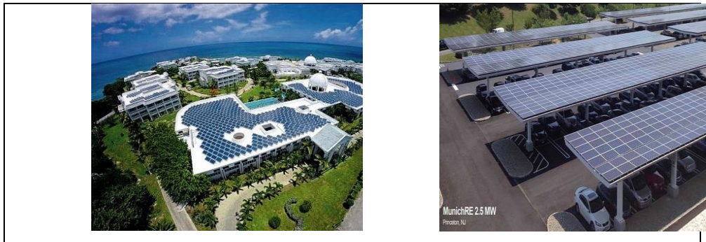
Figure 6: Examples of Building-integrated photovoltaic (BIPV) systems
