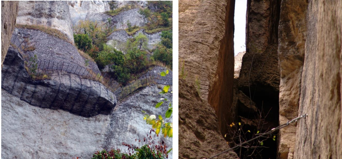
Photo 10: Fortifying with the help of steel ropes and wedges.
