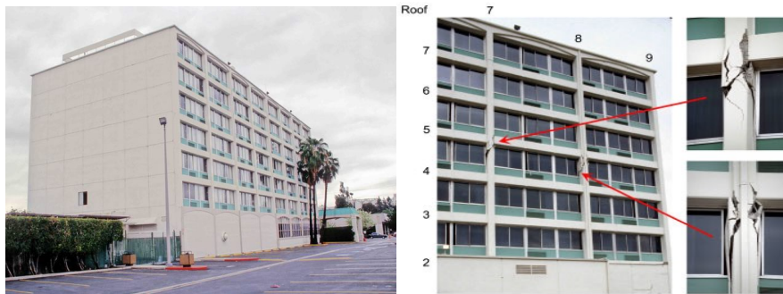
Figure 2. View of the hotel “Holiday Inn” Nuys from North-East Figure 3. Post-earthquake view of in Van Nuys damaged columns
