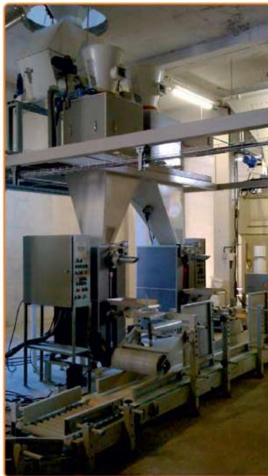
Fig. 5 Bag Filling machines in mill factory Kulpin, Serbia
